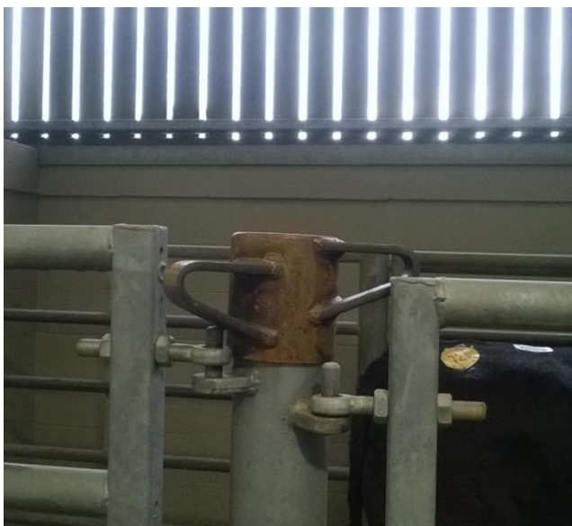
Figure 5.5 Moveable post-topper socket, providing protection from jumping injuries for cattle in a UK livestock market.
