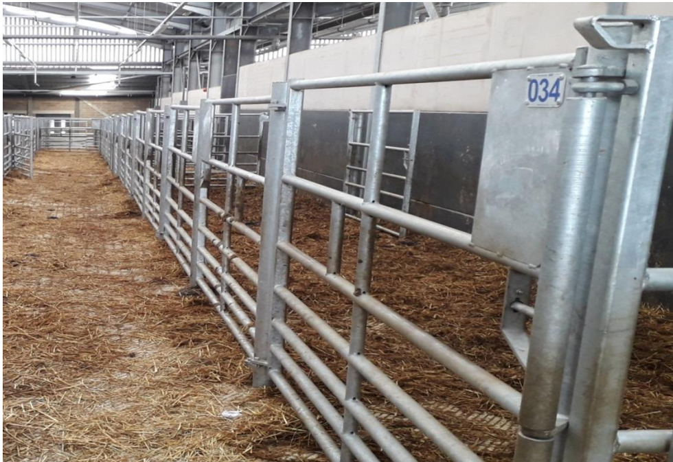
Figure 5.6 Corner of gangways in a UK market. Note the roller bar on gatepost.
