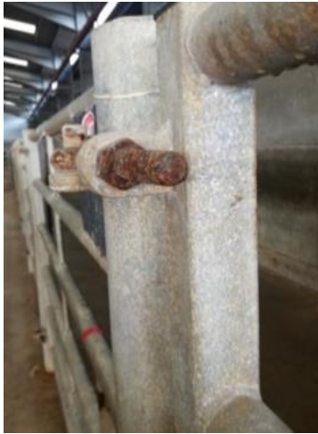
Figure 4.2.4 Protruding bolt which is a risk for contact or bruising in a UK cattle market.
