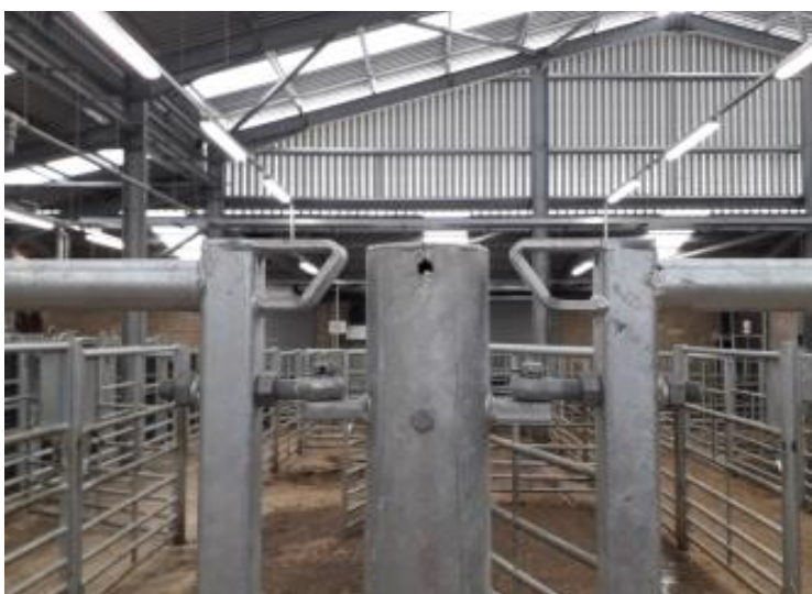
Figure 4.2.2 An example of built-in protection from jumping injuries for adult cattle in a UK livestock market.
