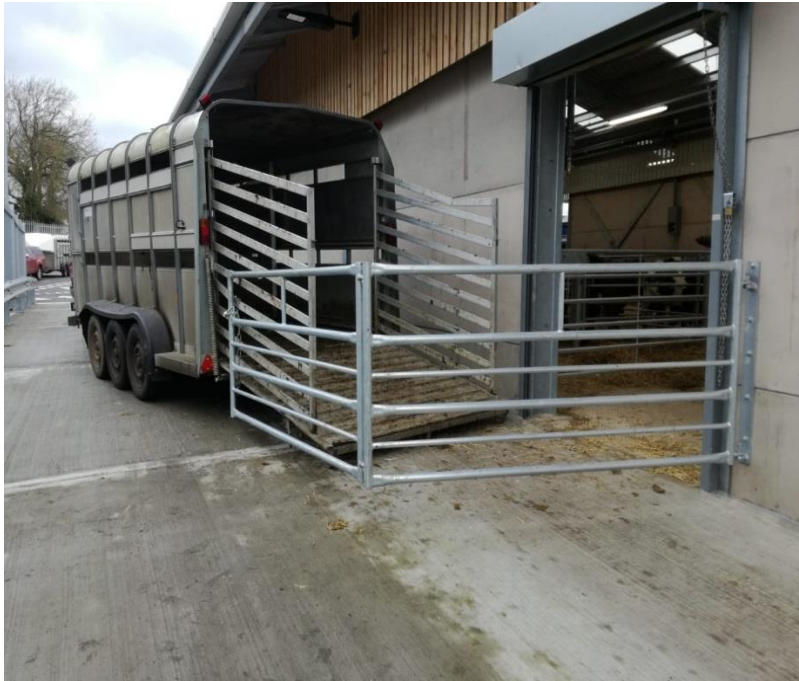
Figure 5.3 Wrap-round, calf loading gate installed in a UK market.
