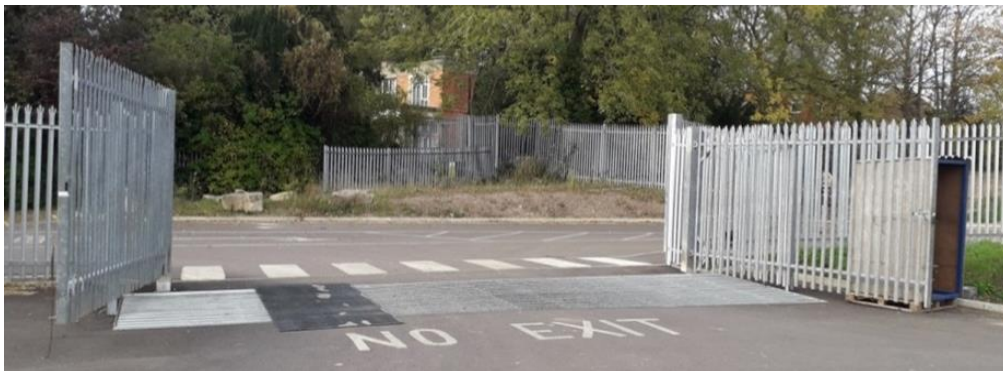
Figure 4.2.3 An example of escape prevention (cattle grid) in a UK market.
