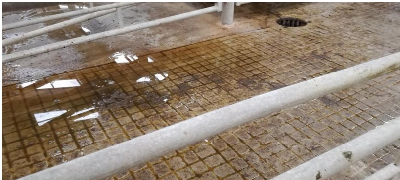
Figure 4.2.6 An example of flooring in a modern UK livestock market.
