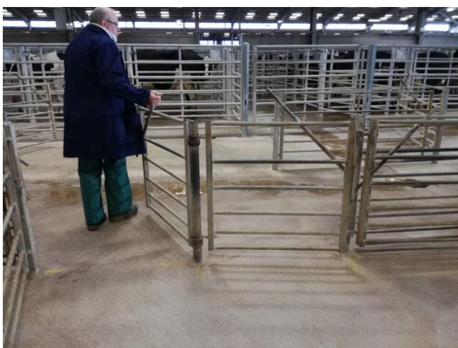
Figure 5.2 Variation of the Poldenvale 360° gate installed in a UK market.
